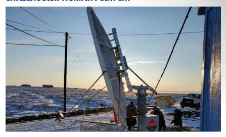
ASTAC recently performed maintenance on its satellite dish in Point Lay to not only raise the dish by 2 feet to reduce snow accumulation, but also in an effort to improve the quality and strength of the satellite signal for both wireless and Internet service into Point Lay.
