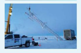
ASTAC dismantled and removed its 17-year old, 200-foot guyed tower near Tarn Road (east of Kuparuk) in January. Crews did an incredible job working in -15-degree temps to safely lower the tower and haul it off site in 40' segments. In May of 2018, a new 200' self-supporting lattice tower was erected allowing ASTAC to continue providing reliable 4G service to the area.
